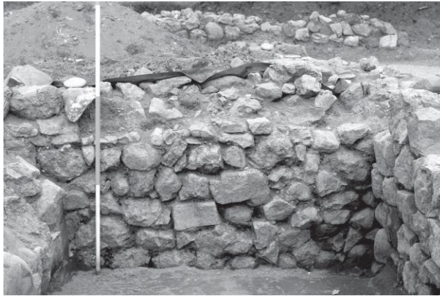
Fig. 8. Gonio (Sector NO 01, Square 97). The face of wall W2 (view from the west). Visible ventilation hole secondarily blinded with an additional stone.
